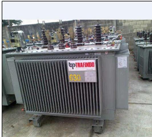
Gambar 3.3 Transformator Distribusi fasa tiga
