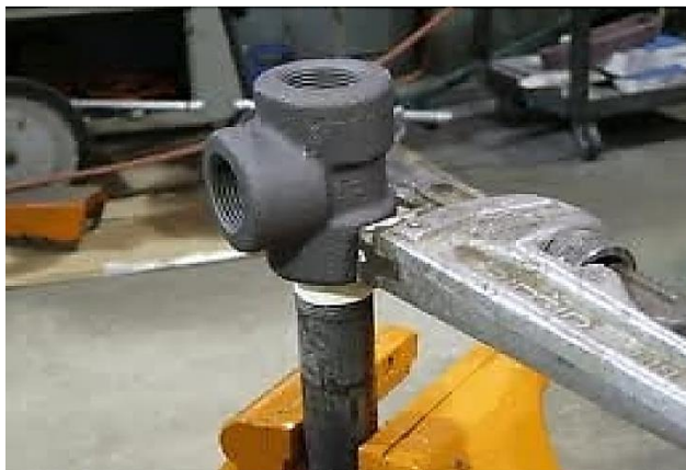
Gambar 2.9 Pasang fitting (socket/elbow/nipple)
